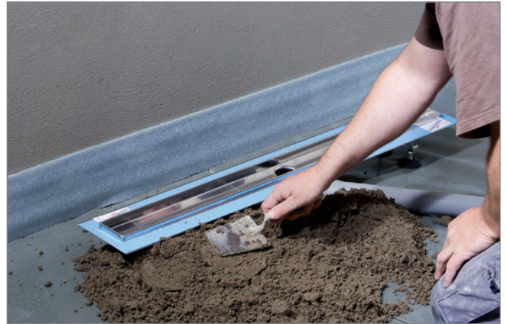
6. Estrich (ohne Hohlräume) einbringen Put in composition floor (without hollow spaces)
